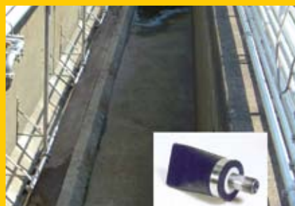
Multiple assemblies installed along one side of the channel produce a single roll mix, keeping solids in suspension.
